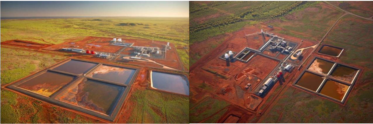
Figure 17-1: Devil Creek Gas Plant, south of Karratha
