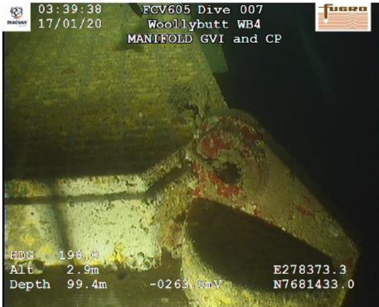
Figure 3-10: WB4 manifold NW roof padeye
