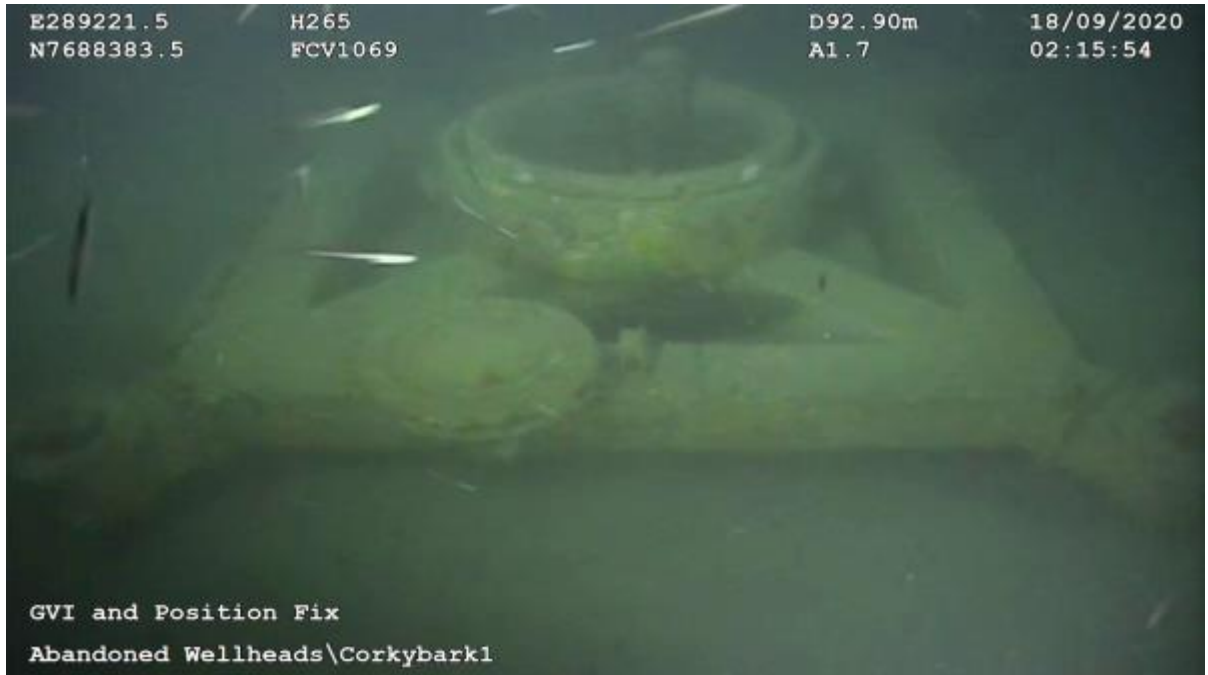
Figure 3-5: CB1 conductor pipe and guide base
