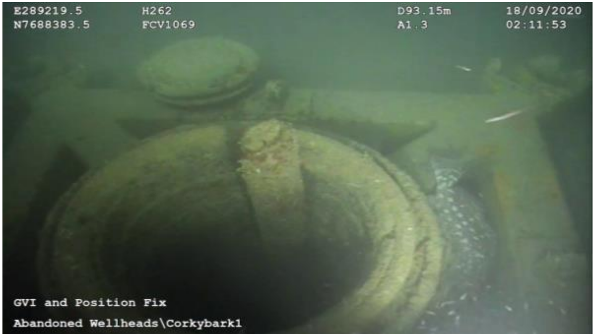
Figure 3-7: CB1 drill string inside conductor pipe on NW side
