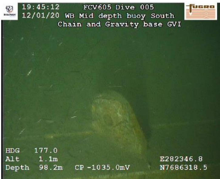
Figure 3-22: South MDB gravity base padeye
