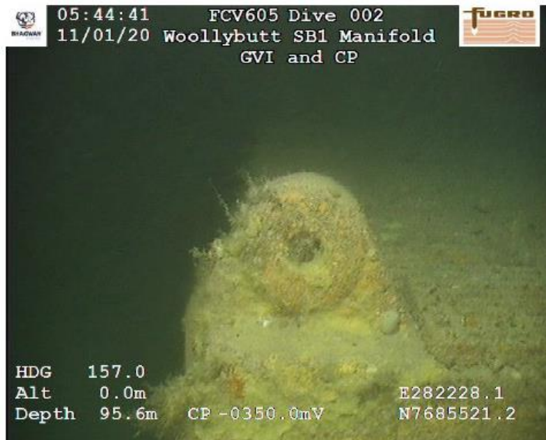
Figure 3-9: SB1 manifold roof padeye
