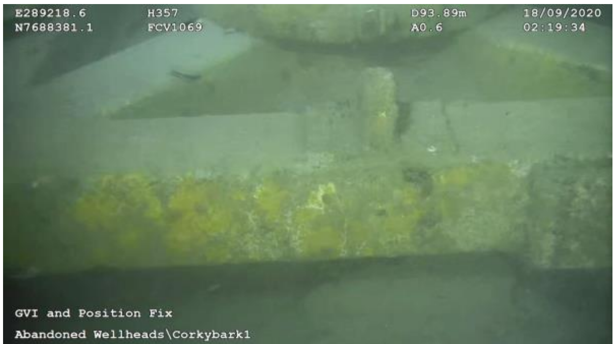
Figure 3-5: CB1 conductor pipe and guide base
