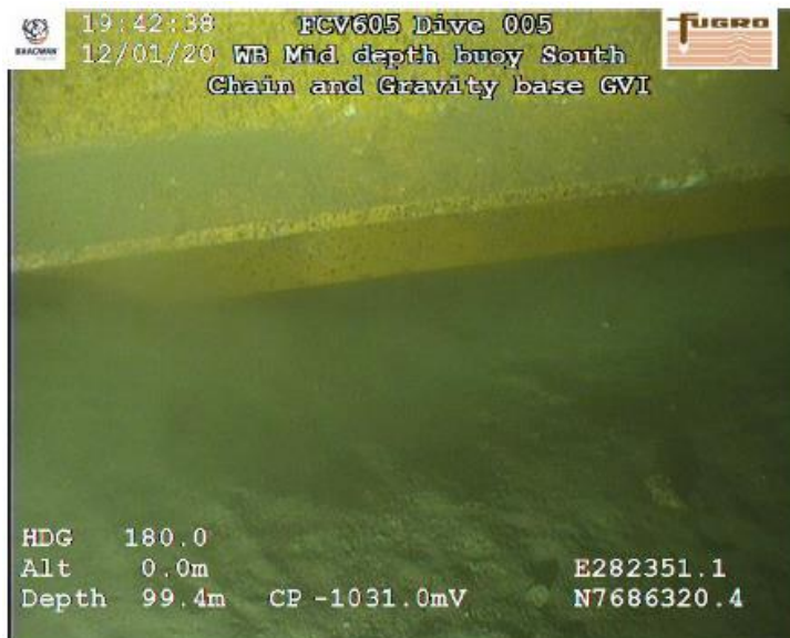
Figure 3-20: South gravity base scour on north side
