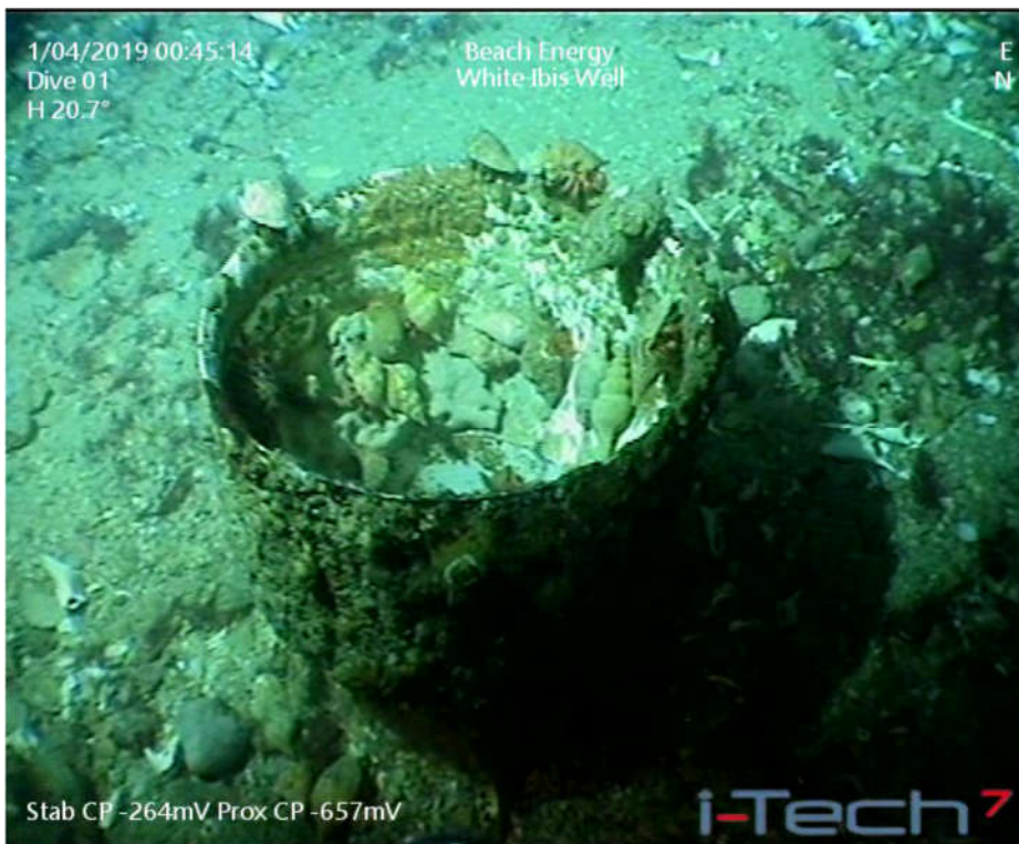
Photo 3.2. Close-up of the White Ibis-1 corrosion cap receptacle
