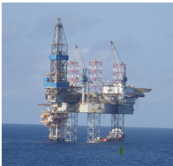
Figure 2-2: Positioning the MODU alongside a Wellhead Platform
