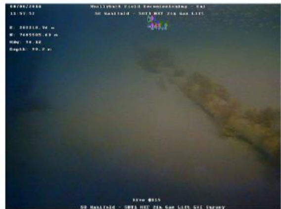
Image 2.6-04 - 2" Gas Lift - Free Span
