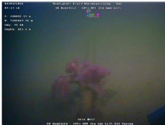
Image 2.6-03 - 2" Gas Lift - Marine growth
