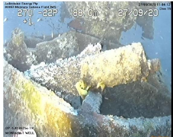
Figure 2-1: Images of Montara-1 wellhead – debris cap (top left), TGB (top right, middle left), wellhead upper structure (middle right), hose debris and broken guidepost in TGB structure (bottom L-R) (Jadestone Energy, 2020)
