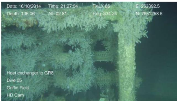
Heat Exchanger to GR8
