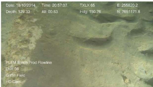
PLEM 8 inch Production Flowline
