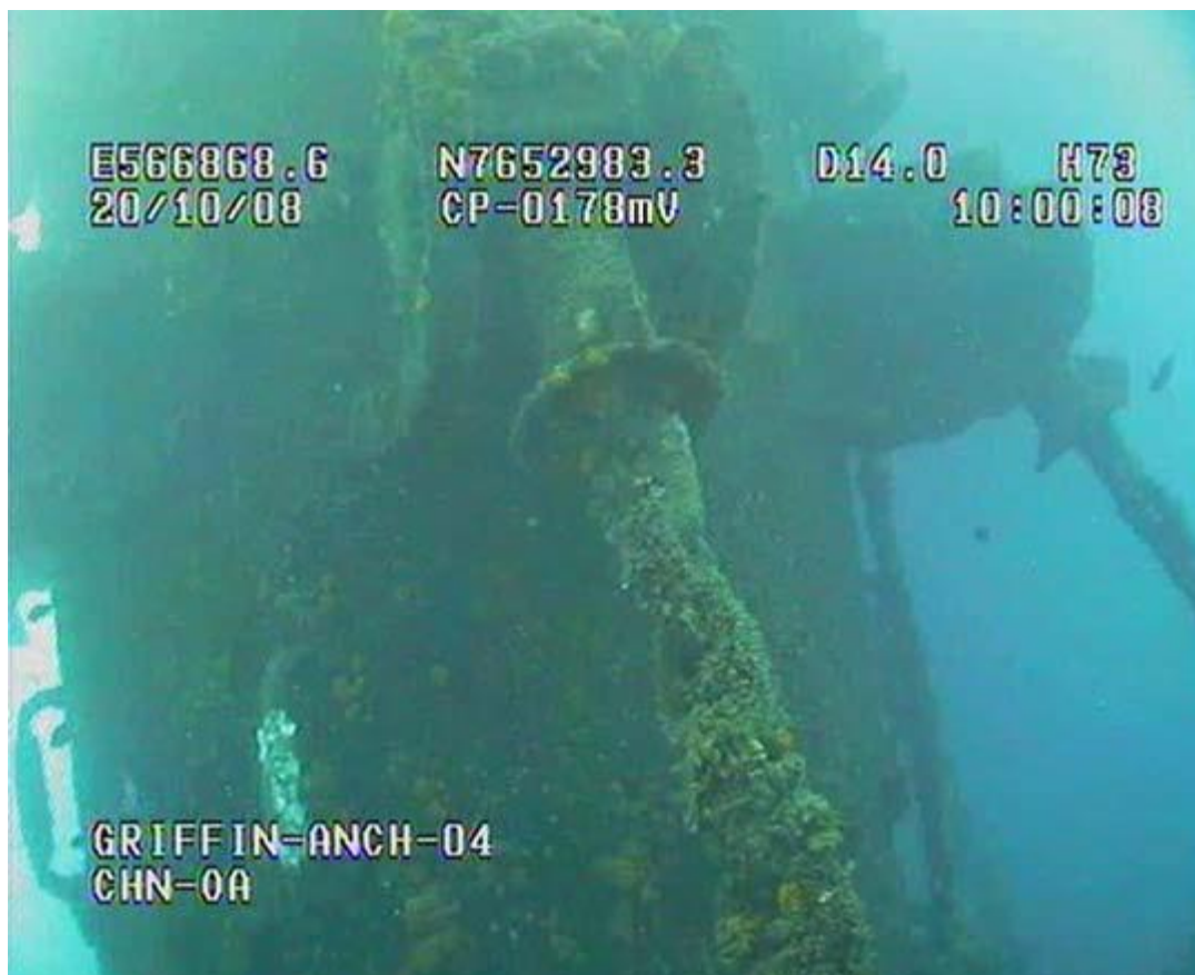
Figure 2-2: Epibiota on the Riser Anchor Chain 4 Within the Griffin Field
