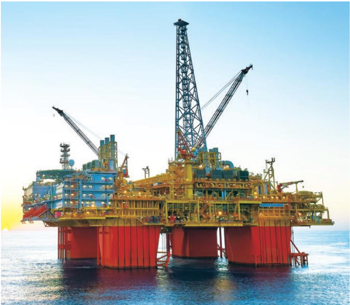
Figure 3-5: The central processing facility (CPF)
