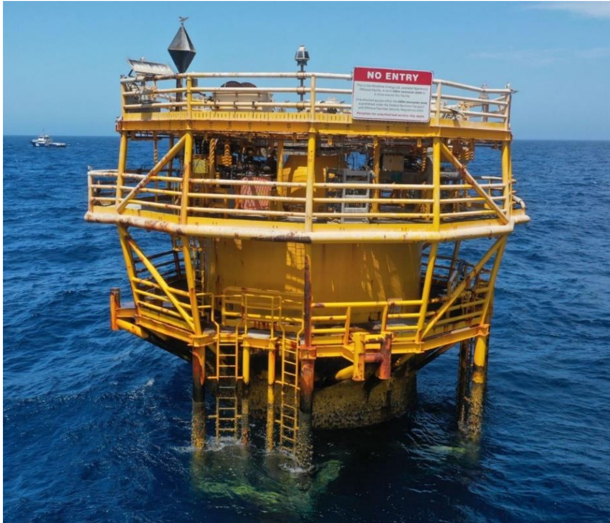
Figure 3-4: Topsides section of the RTM
