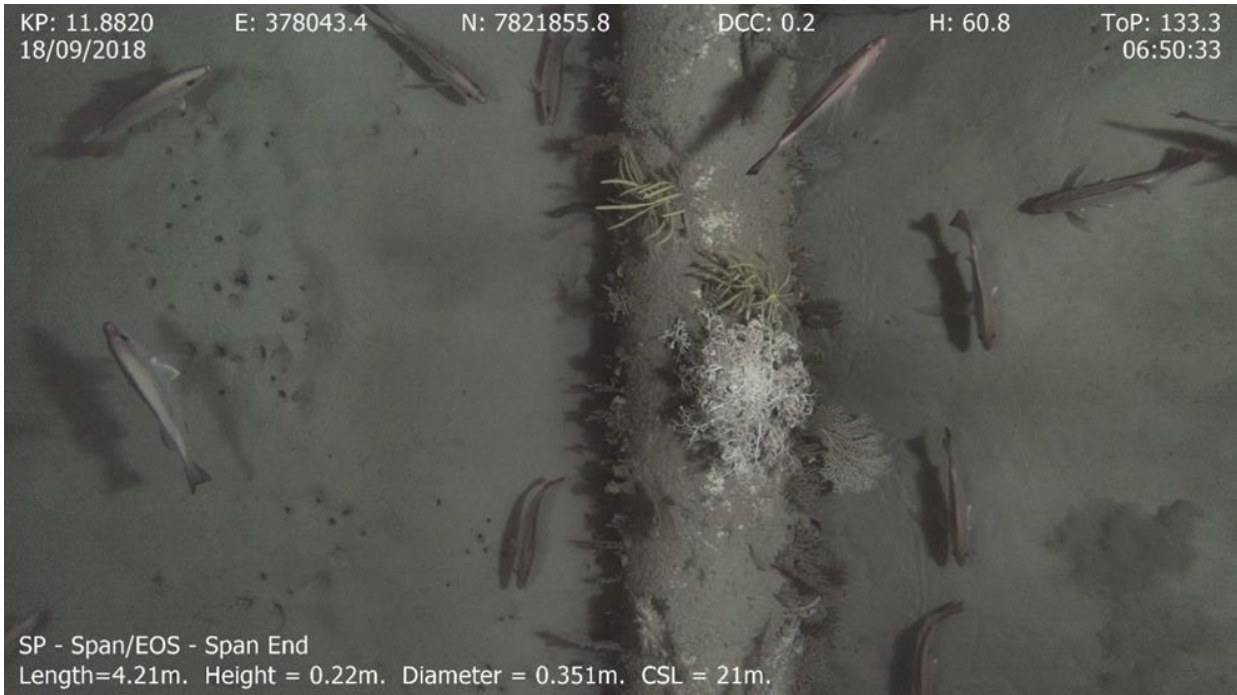
Figure 3-4: Section of the Echo Yodel pipeline in situ
