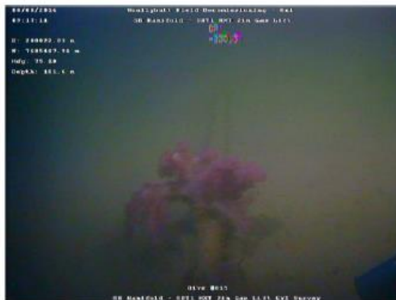
Image 2.6-03 - 2" Gas Lift - Marine growth
