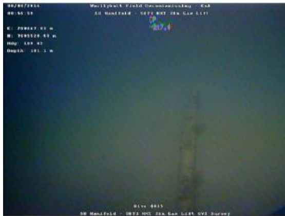
Image 2.6-01 - 2" Gas Lift - Exposed
