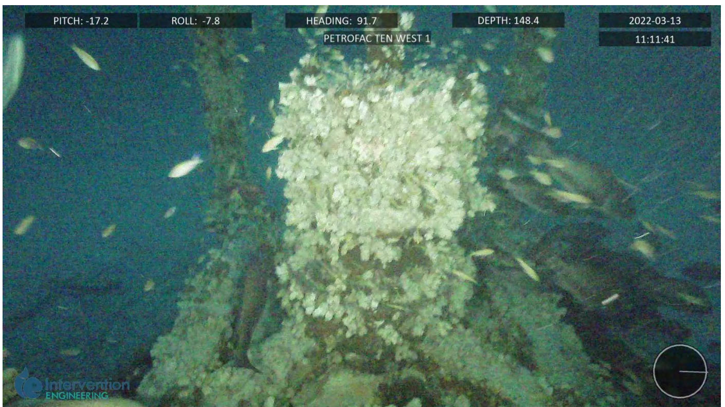
Figure 5 Ten West 1 corrosion cap
