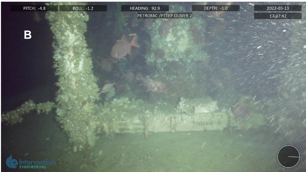
Figure 5-2: Oliver-2 wellhead: A – view of the top of the wellhead including guide posts and corrosion cap; B – permanent guide base at seabed level
