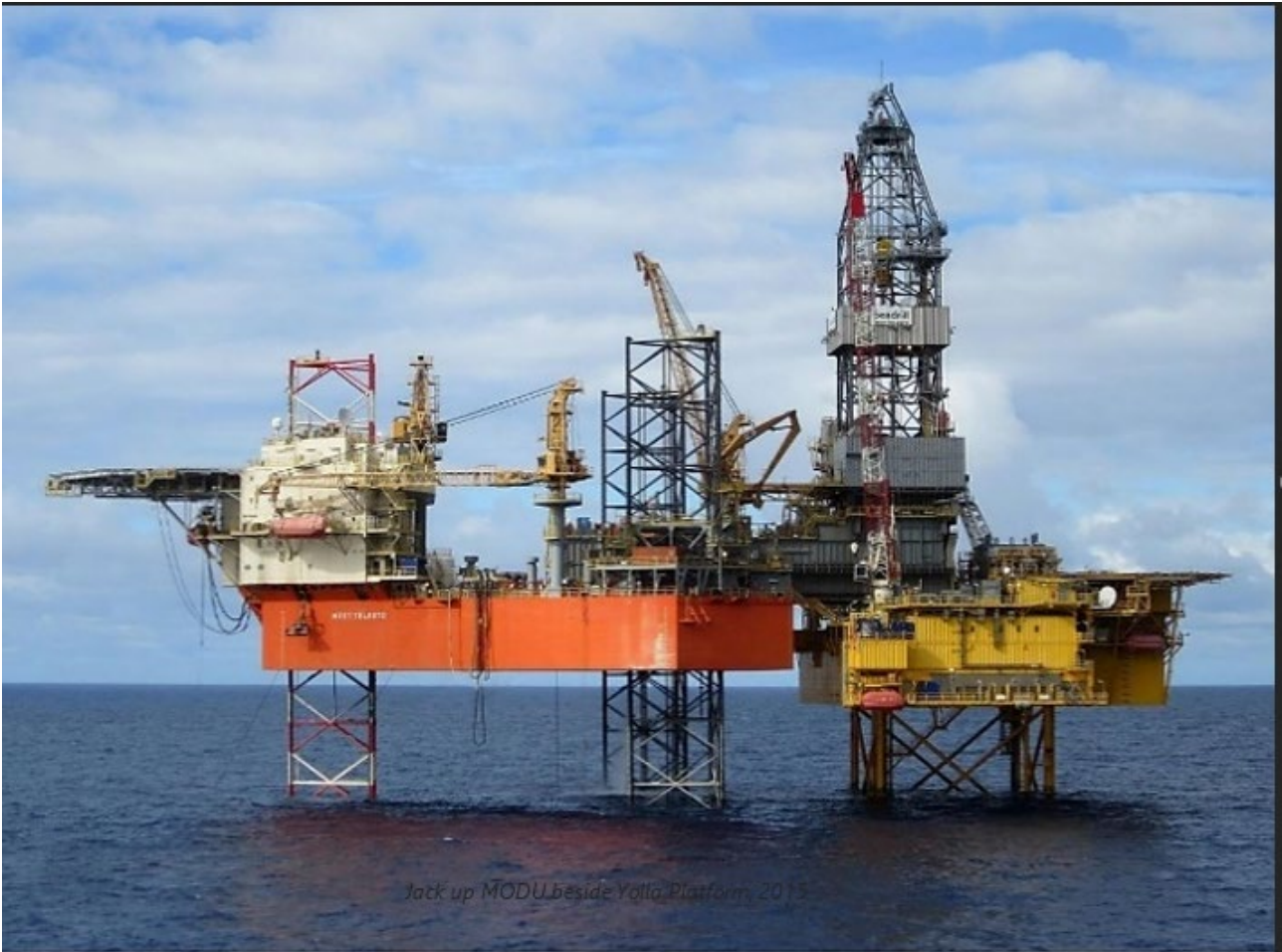
Figure 4-3 Previous Jack-up rig work on the Yolla-A platform
