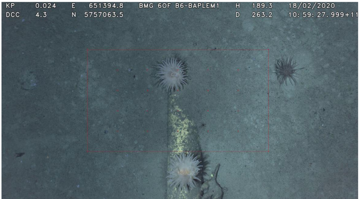
Figure 6-1 Image from 2020 GVI showing the B6 Oil flowline transitioning from above to below the seabed (Ierodiaconou, et al. 2021)
