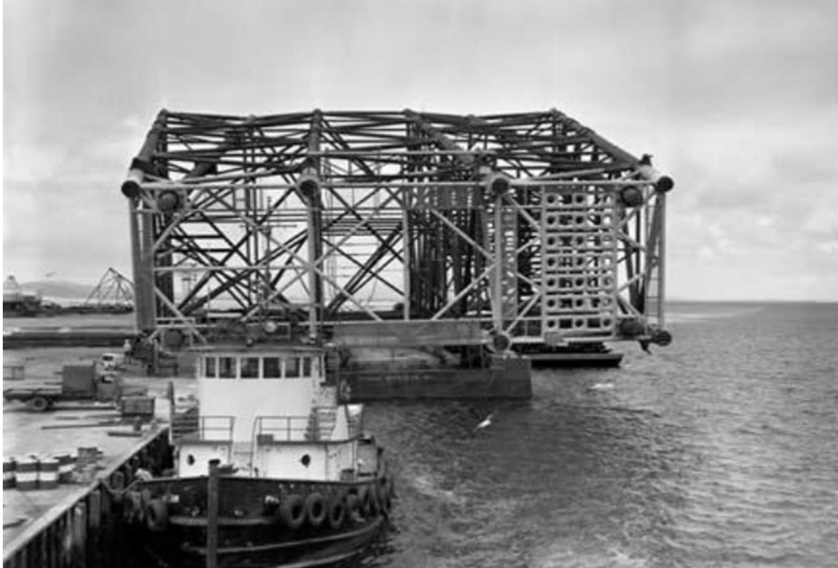
Figure 1-2 One of the Kingfish Steel Piled Jackets being transported to its installation location
