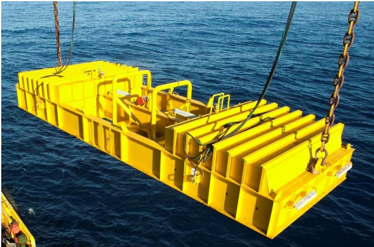
Figure 2-1 MEFF field gravity base during installation (from GHD et al., 2021)
