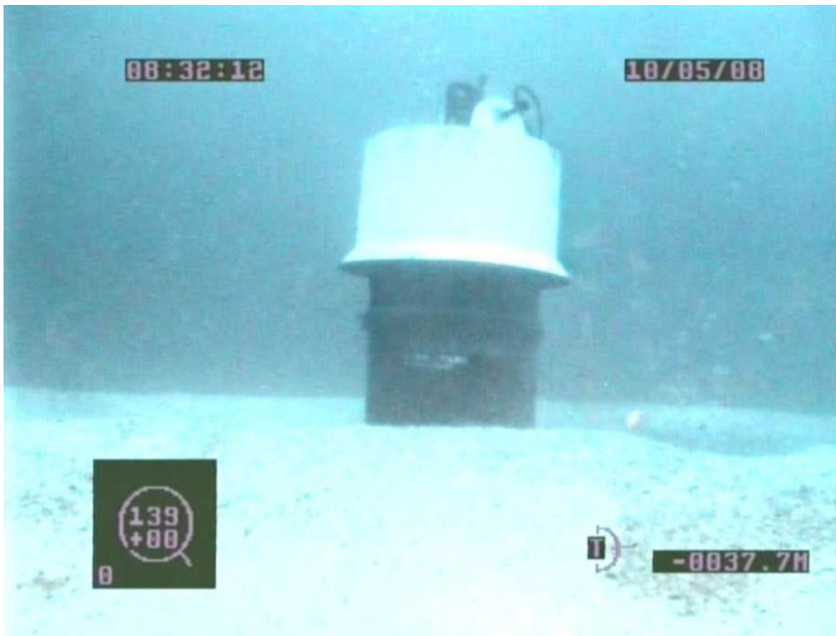
WSH-3 well and temporary abandonment cap
