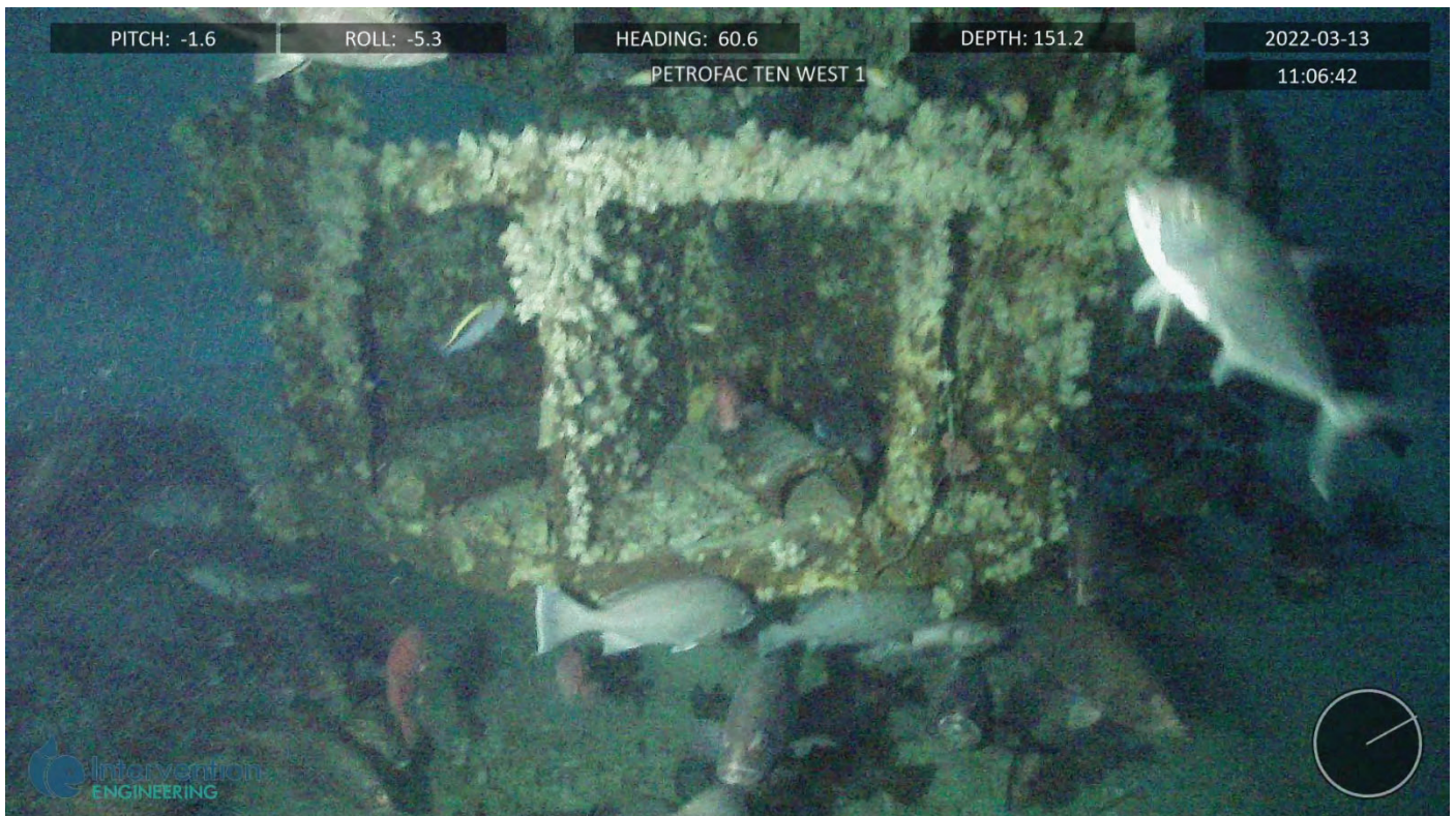
Figure 4 Ten West 1 example of corrosion
