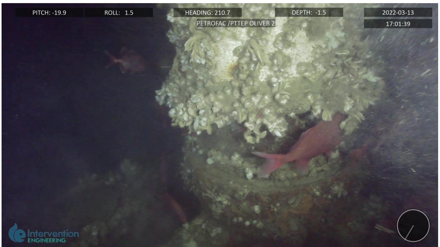
Figure 12 Oliver 2 Example of corrosion on wellhead
