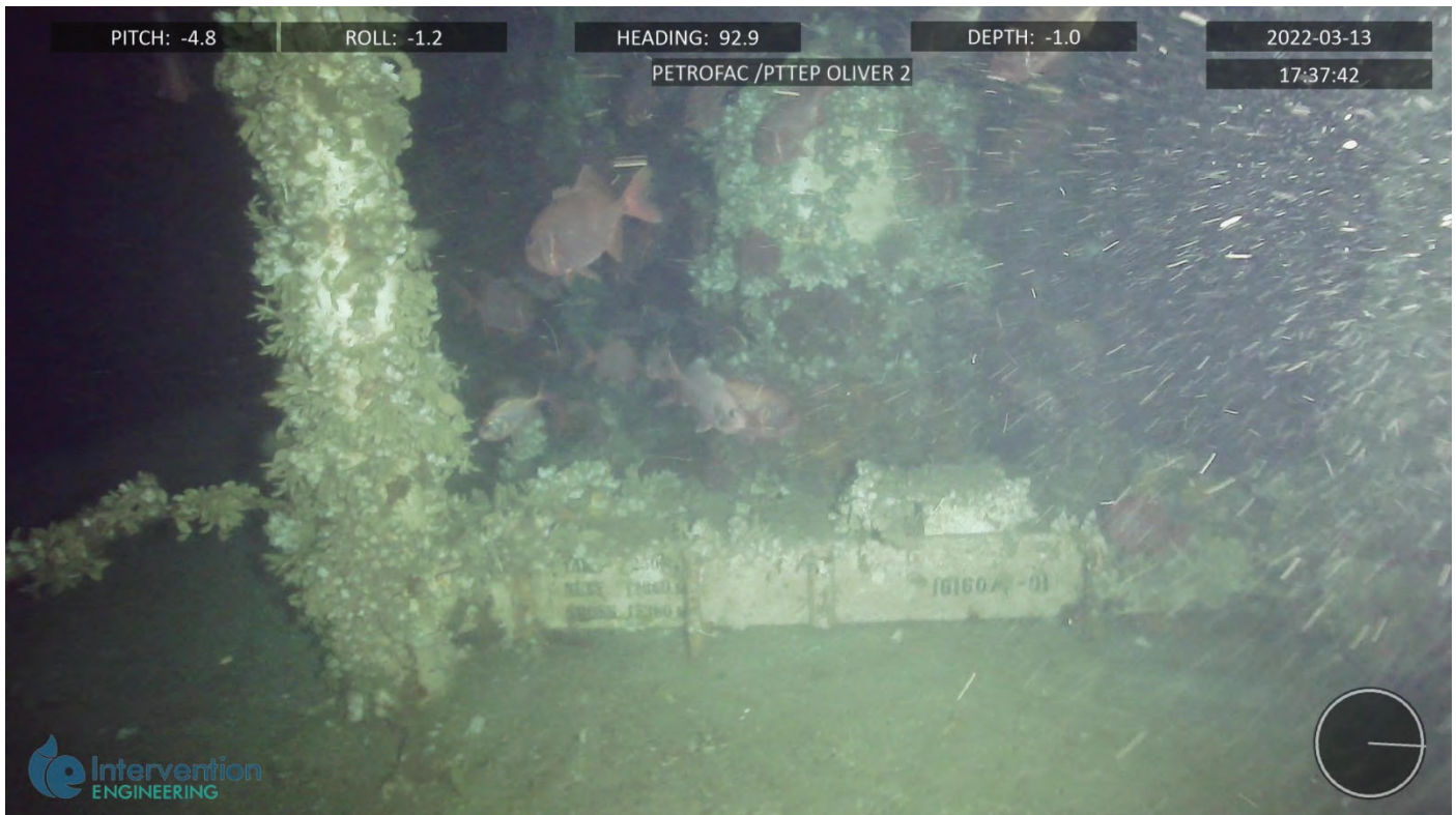
Figure 16 Oliver 2 PGB at seabed level
