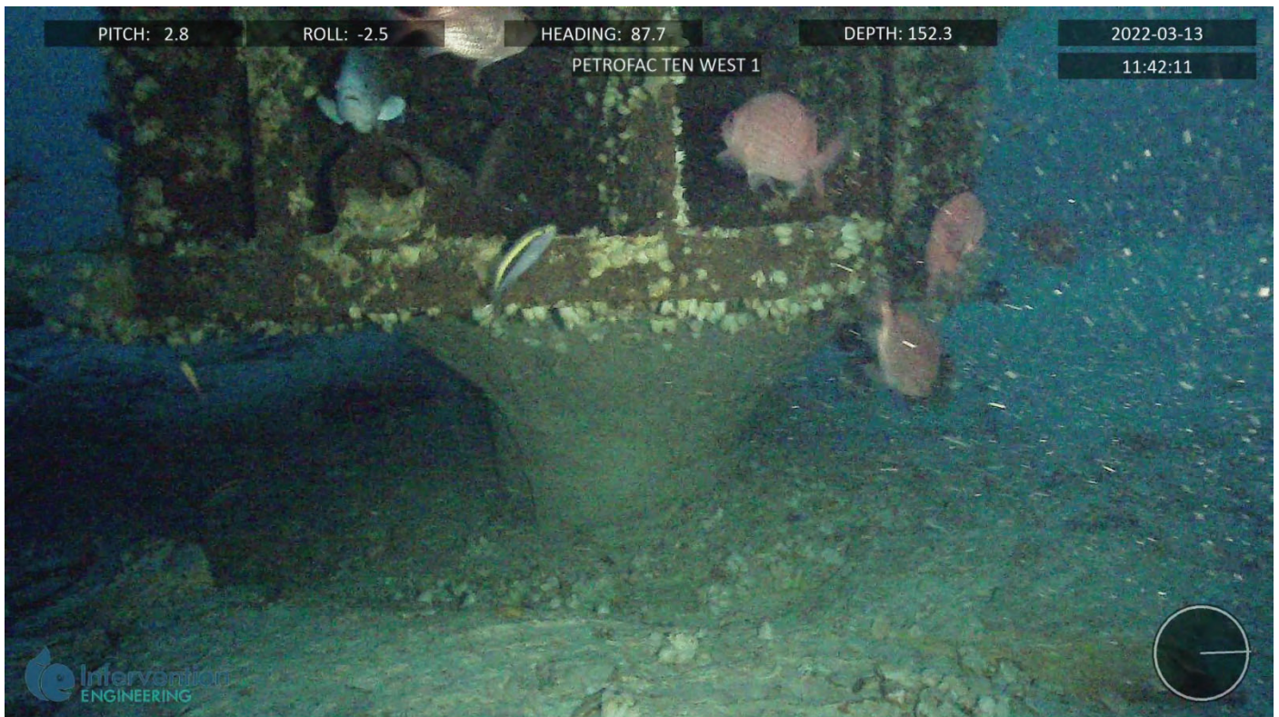
Figure 6 Ten West 1 example scour under guide base.
