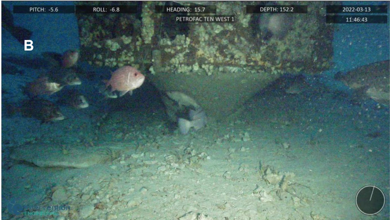
Figure 5-3: Tenacious West-1 ST1 wellhead: A - view of the top of the wellhead including guide posts and corrosion cap; B - view of scour under the temporary guide base and sign of cement returns
