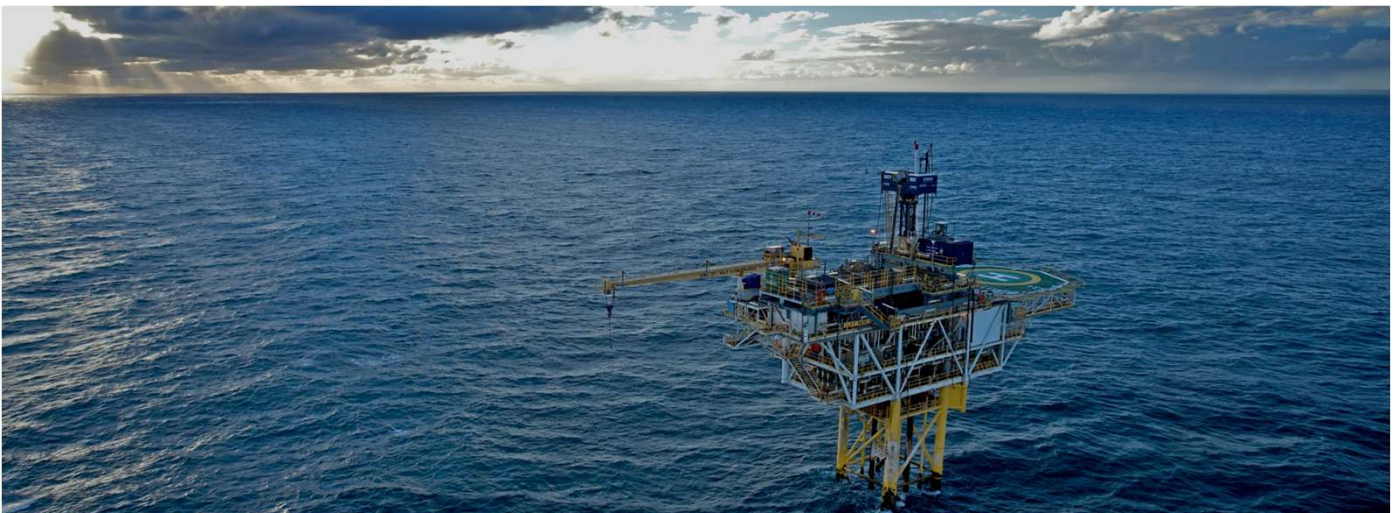
FIGURE 1. Cliff Head Alpha Offshore Platform
