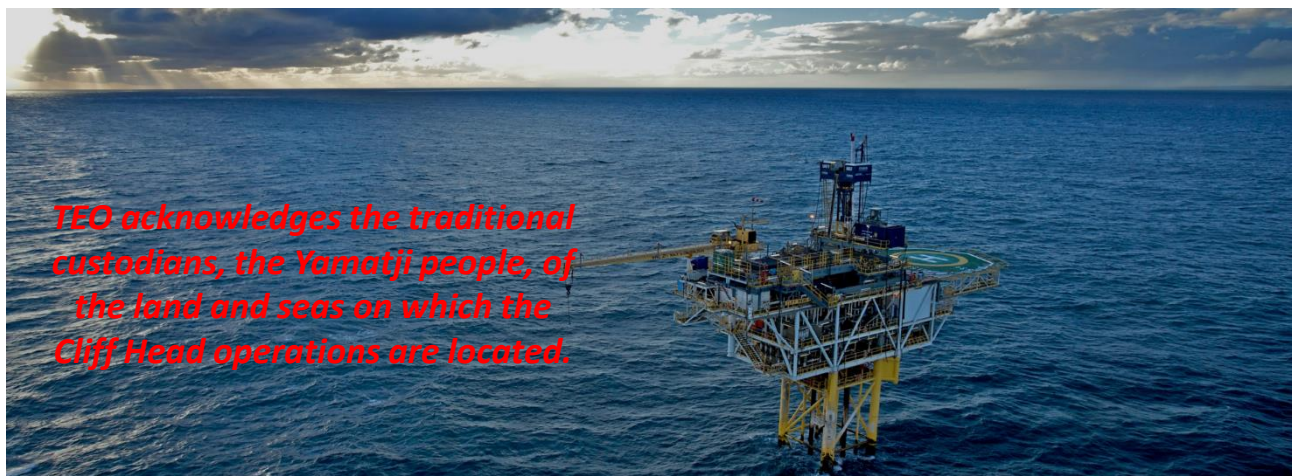
FIGURE 1. Cliff Head Alpha Offshore Platform
