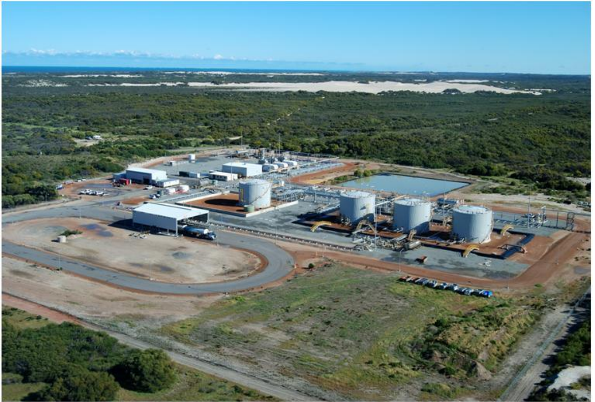
Figure 8-3: Arrowsmith Stabilisation Plant
