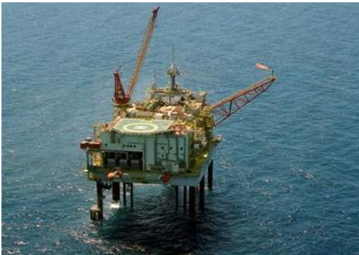
Figure 1-2: Aerial view of Stag Facility
