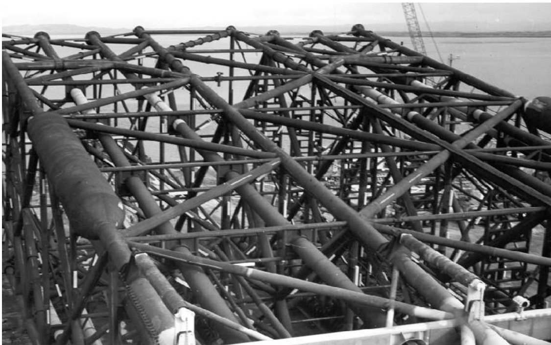
Figure 1-3 The Mackerel Steel Piled Jacket prior to installation, showing the complexity of the structure
