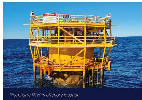
(FPSO) facility, Nganhurra RTM
