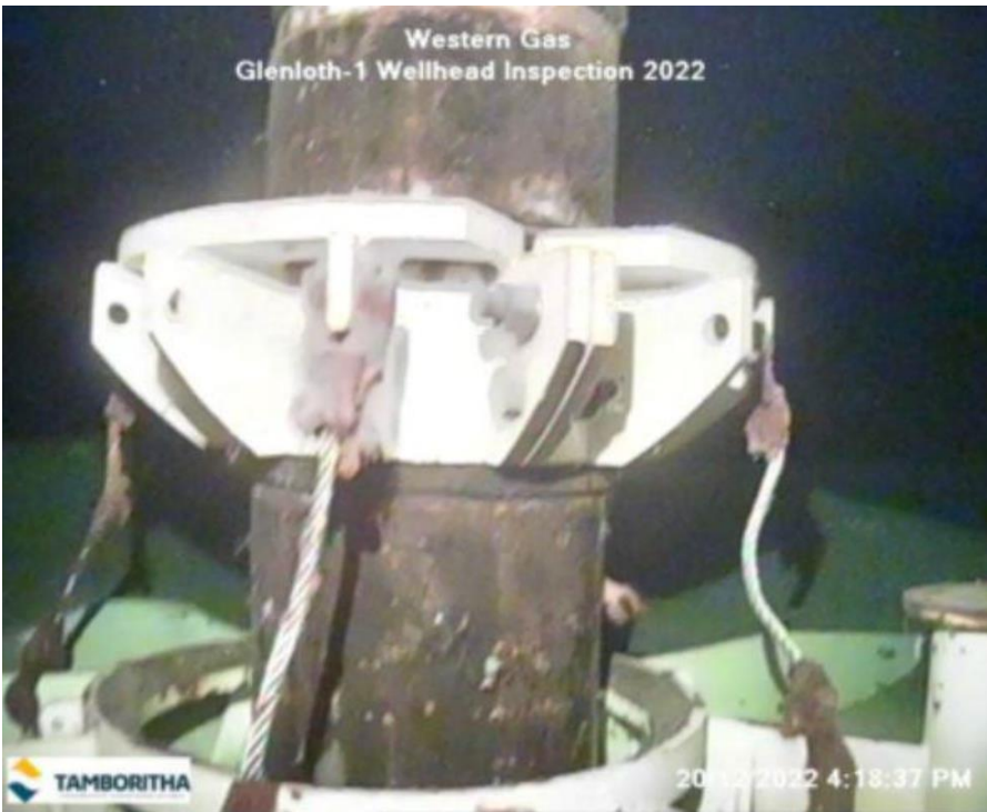
Figure 2-5: Photograph of the Glenloth-1 guide base connection to wellhead
