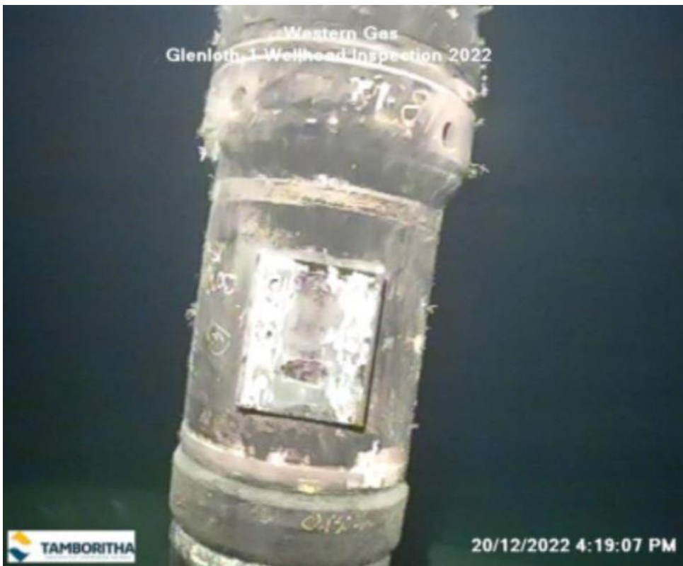
Figure 2-4: Photograph of the Glenloth-1 well conductor
