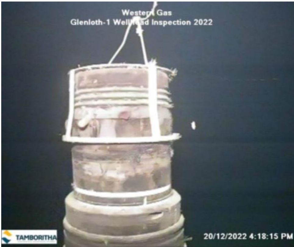
Figure 2-3: Photograph of the Glenloth-1 well conductor debris cap
