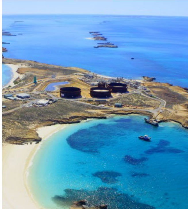
Varanus Island Gas Plant
