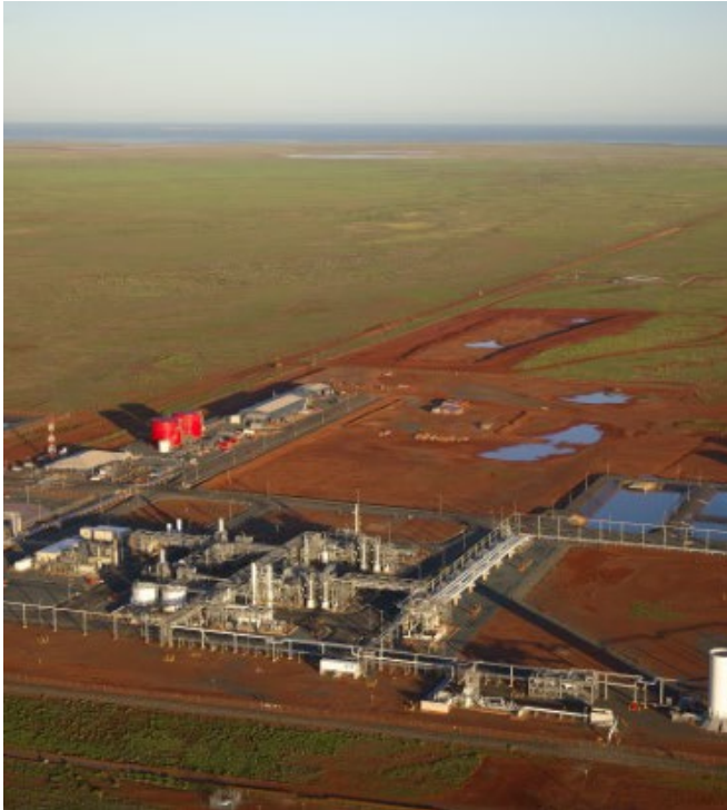
Devil Creek Gas Plant
